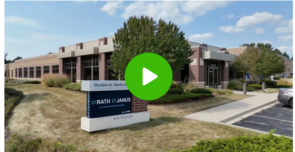
Avire US installed 125kW of solar panels at their Rath Communications facility in Wisconsin. The panels are expected to provide for 98% of power demand during summer months. (Picture credit: Rath Communications)
