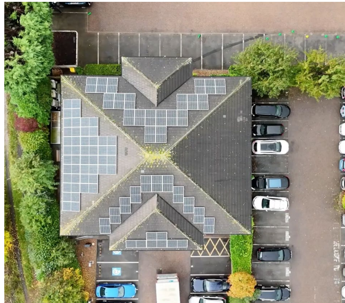
Ramtech's new solar panels (Picture credit: Ramtech)
