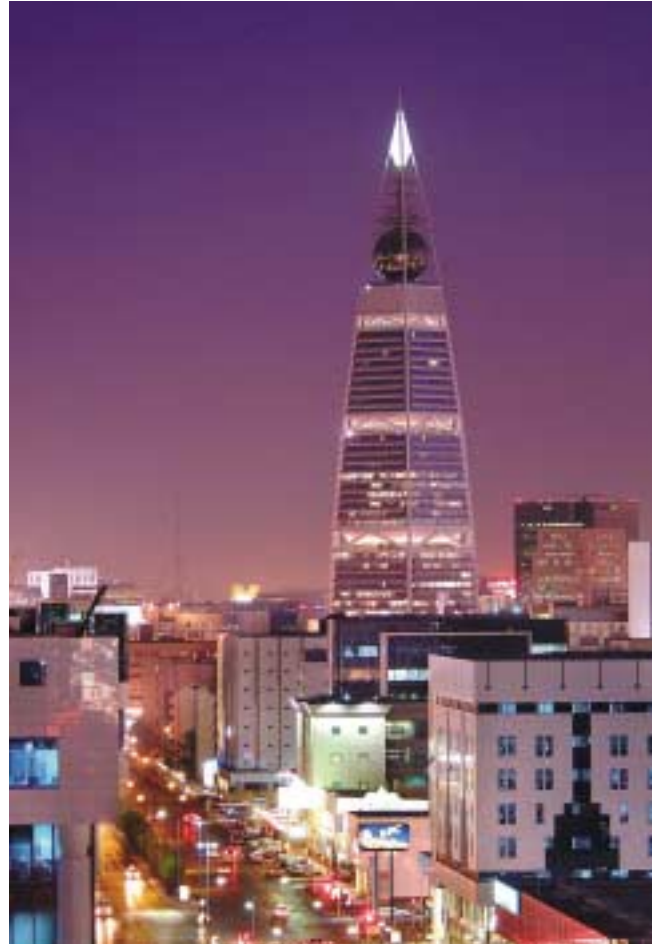
The Al Faisaliah hotel and office complex in Riyadh, Saudi Arabia, where E-Motive LCD information displays are fitted in the elevators.
