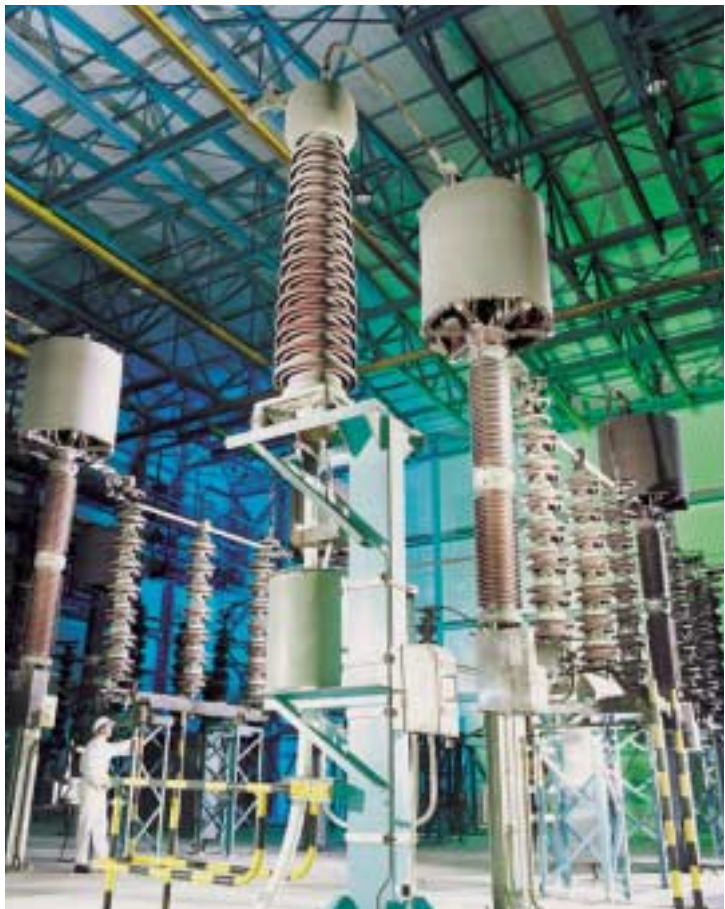
In the UK, the National Grid Company specifies Cressall resistors to protect electrical power distribution equipment.
