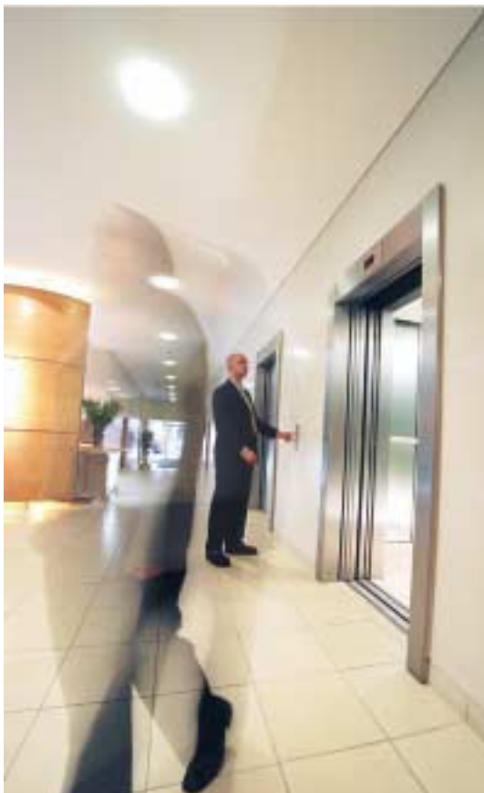
Elevators at the Fountain House offices, in the City of London, are equipped with Memco door safety sensors.
